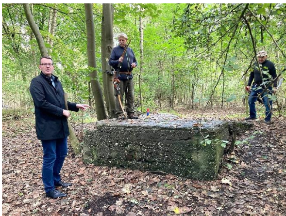
A Concrete Shelter
