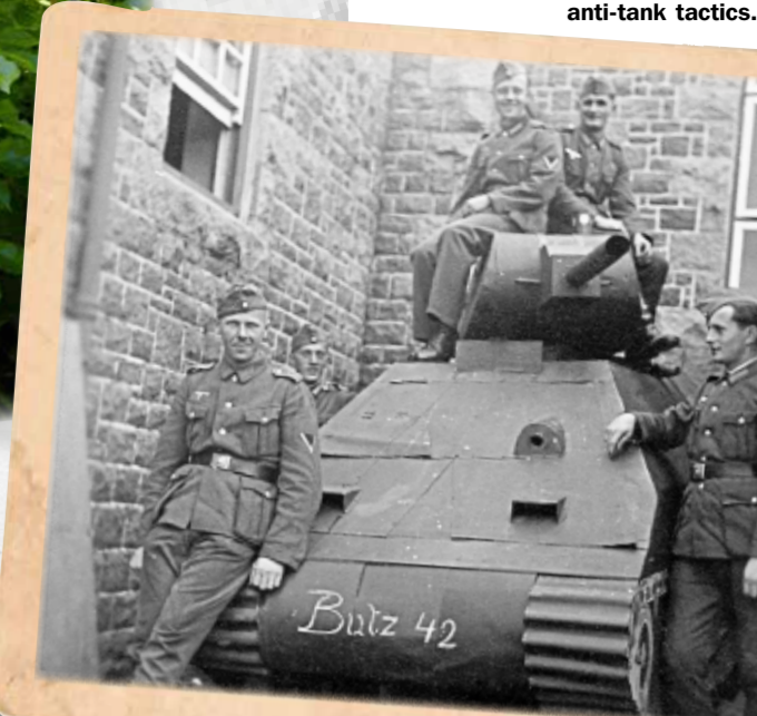
Below: Panzerjäger – quite possibly at the Intermediate School. Dummy tanks like this, which were usually built on a car chassis, were used for training troops in anti-tank tactics.
